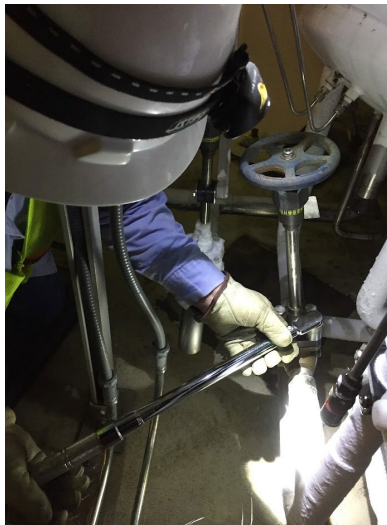
Reassembly of BK9412T applying proper torque with Torque Wrench.
